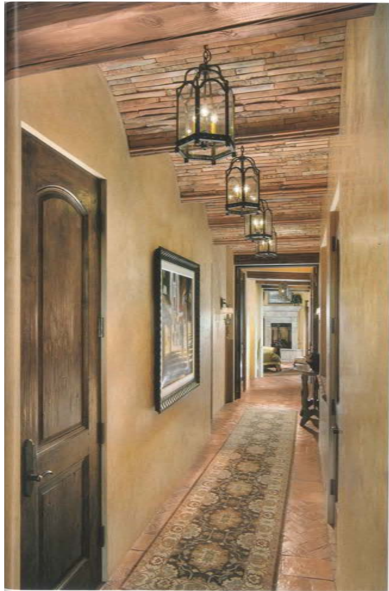
In a hallway leading to the master suite, the ceiling's barrel vaults were made with pieces of tile that were left over from the home's roof. Lanterns are from Steven Handelman Studios in Santa Barbara, California; the rug is by Azadi Fine Rugs.
