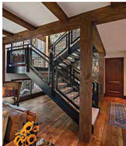
Above Contemporary floating steel staircase with concrete steps, brick inlay landings and metal lattice guard. Top Golf course view of mountain contemporary home with dramatic two-story patio off the great room, and wraparound deck off the master suite. Bottom Street view of mountain contemporary main house and detached garage.
